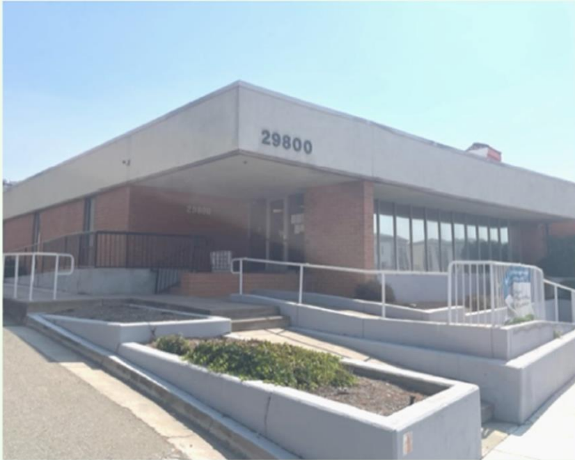
MISSION OFFICE (TENANT OCCUPIED)
